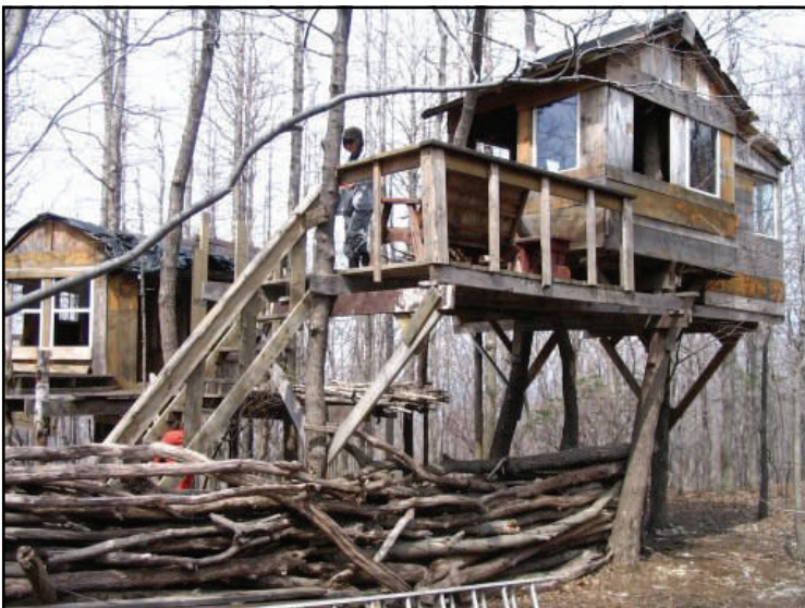
Two of the three illegally constructed structures removed from National Park Service Appalachian Trail corridor land near Little Gap. Photo by Bill Steinmetz.
