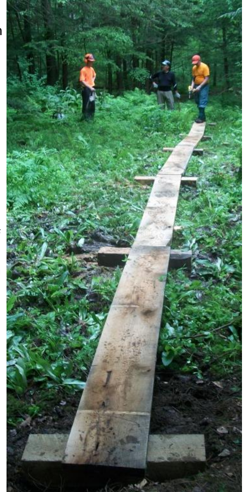
ABOVE: Trail Crew installing "bug" bridging. Courtesy of Daryl Warren
